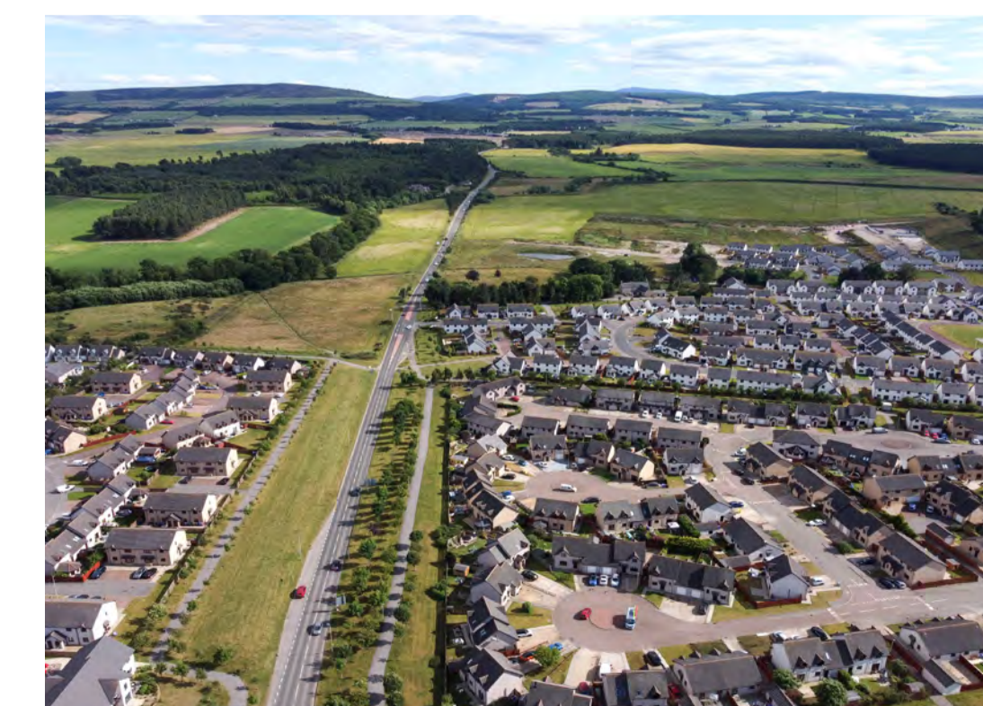
Aerial View Elgin South
