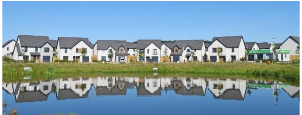
Bertha Park features innovative natural drainage centred on Bertha Loch
